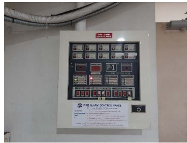
fire alarm control panel
